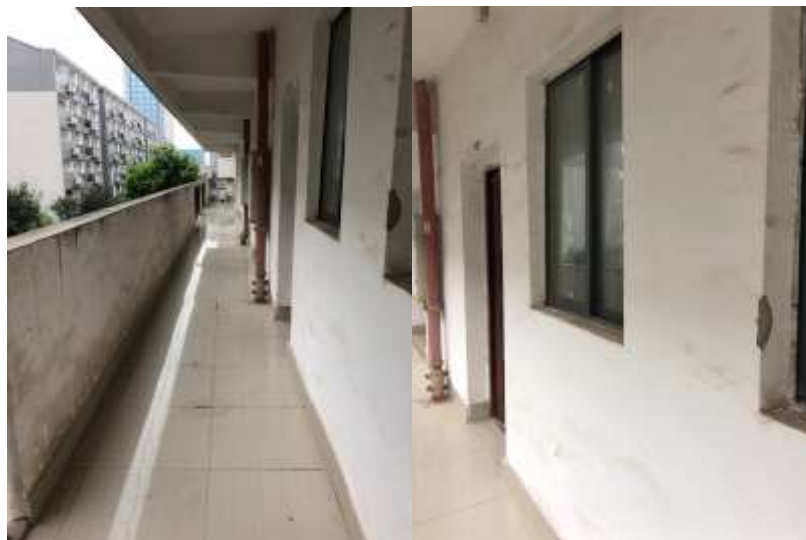
Exterior of the dormitory
