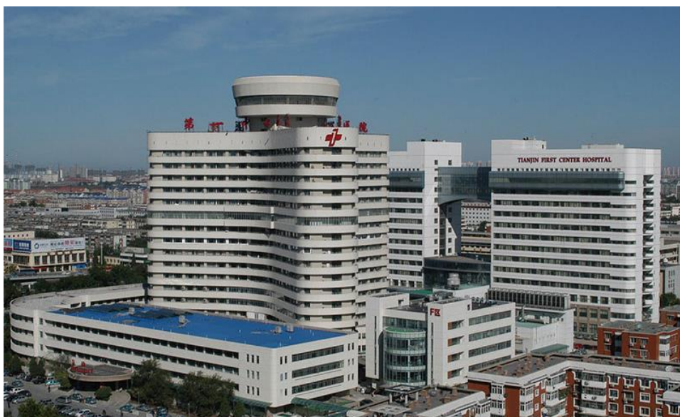
Tianjin First Central Hospital established its Oriental Organ Transplant Center in 1998 with an investment of less than 20,000 RMB. The center broke ground in 2002 on its new 17-story building with 500 transplant beds. The Tianjin municipal government provided about 25,000,000 RMB in funding, aiming to build Asia’s largest integrated organ transplant center.
