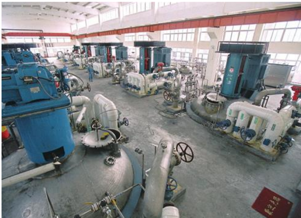
An immunosuppressants manufacture plant
